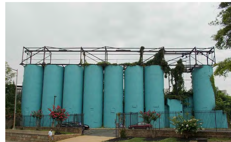
J. Silos on Rhode Island Ave.
