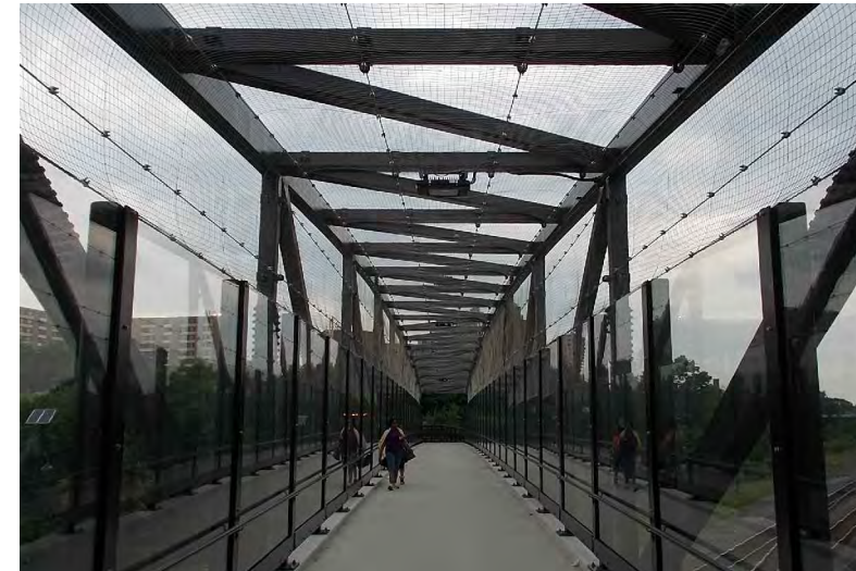
F. Metro Bridge
