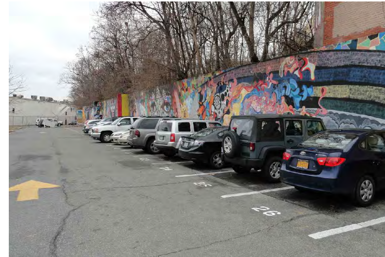
F. Retaining wall
